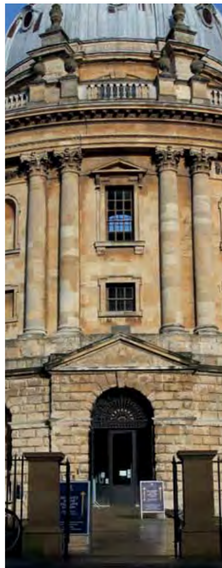
The new Radcliffe Camera entrance
