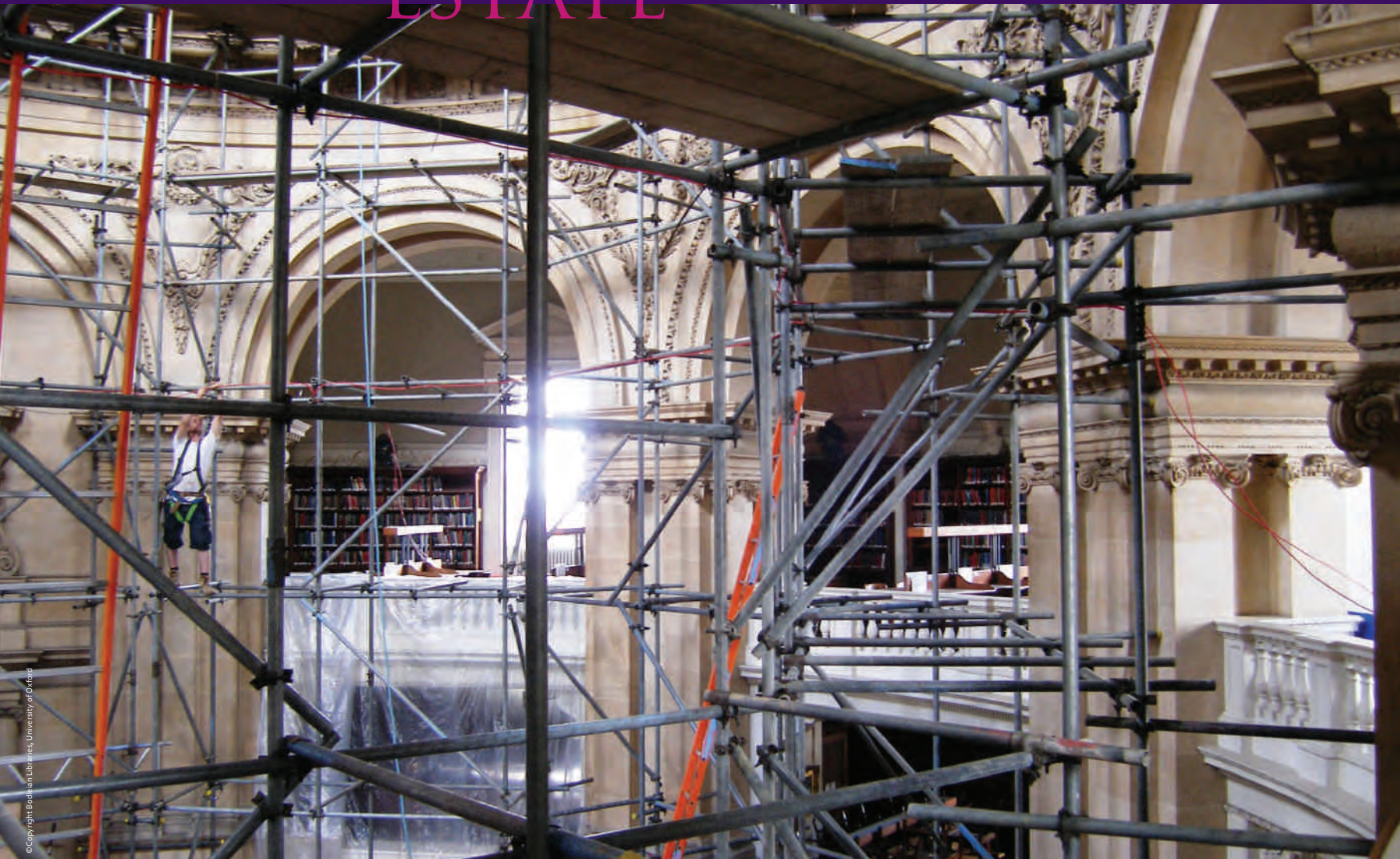
Scaffolding in the Radcliffe Camera upper reading room
